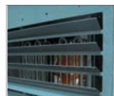
Detalle deflectores. View of deflectors.
